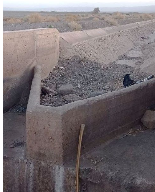
Fig. 1 Duckbill Spillway located in the Bam irrigation network - Kerman Province
